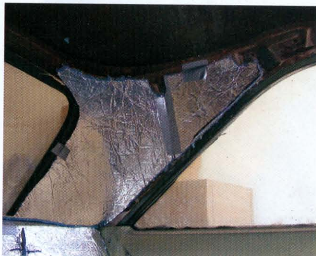
9 Even smaller areas, such as this rear corner of the roof, should be insulated.
